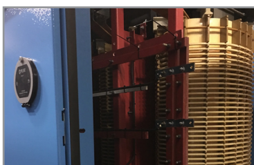
Infrared viewing window & custom enclosure finish
